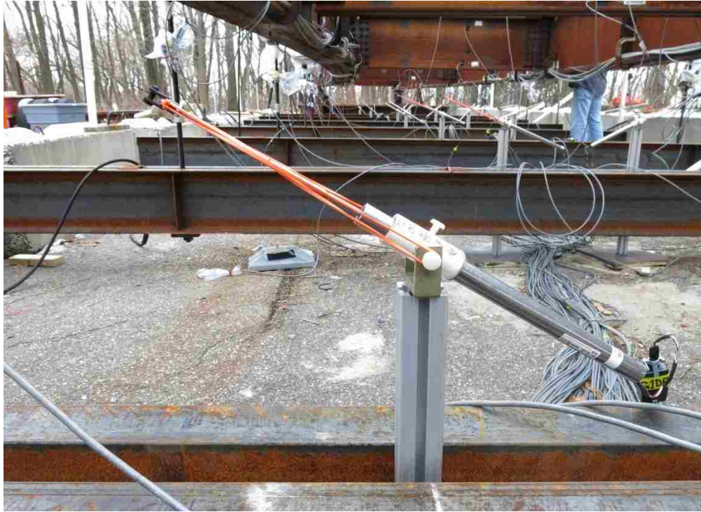
(c) LVDT to measure displacements of intermediate point installed on extruded aluminum bar stand
