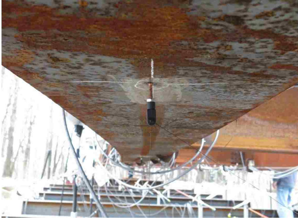
(a) Intermediate target point located 1 in. below the bottom flange
