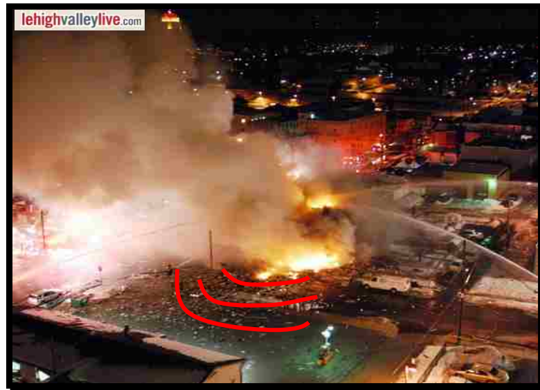
Figure 19 Fragments distribution around the demolished house [5].
