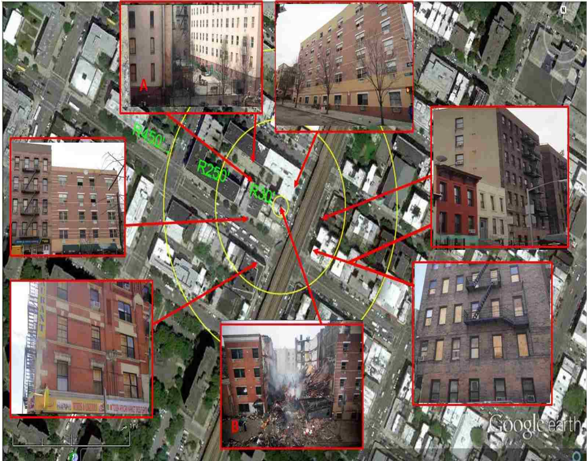
Figure 41 Associated damage between 30 to 250 ft [9]
