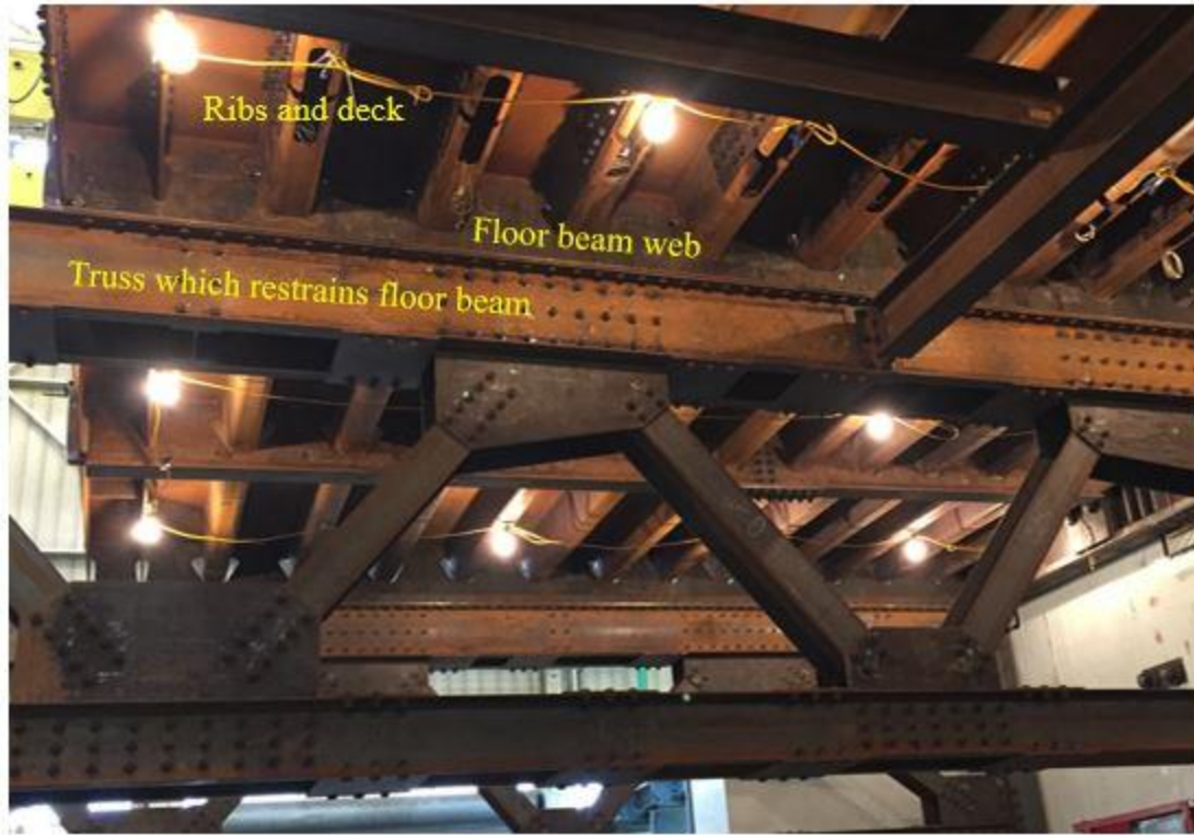
Figure 3. Photo. SOBD floor beam attached to transverse truss. Source: Joseph Saunders.
