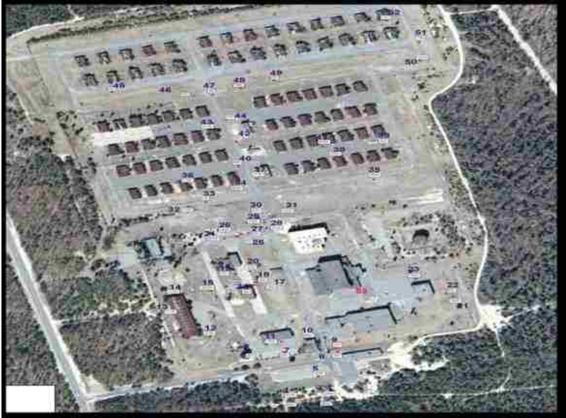
Figure 2. Pre-2002 aerial view of the BOMARC site provided by Cabrera Services. Note the white patch in the upper left hand corner, the concrete poured to cover the affected area and shelter 204 (roof missing), the site of the fire.
