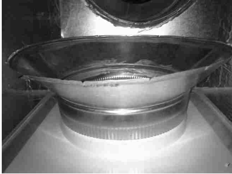
Figure 3. Diffuser inlet configuration.
