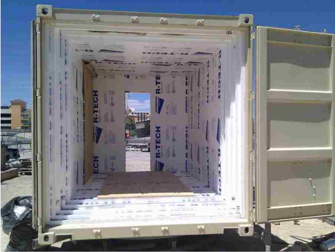
Figure 7 - Insulation Installation in the Facility
