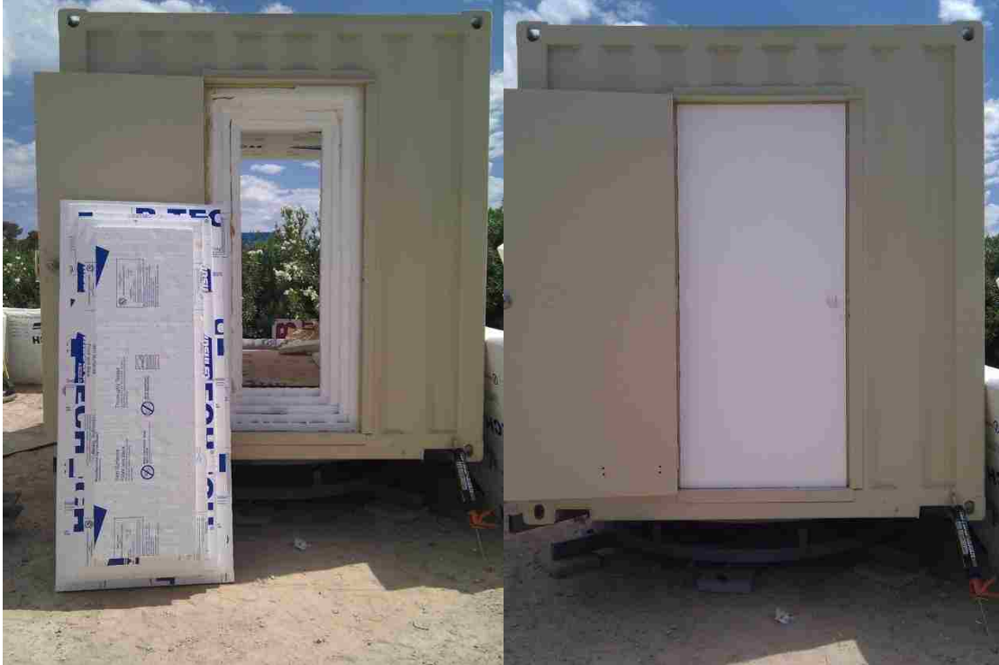
Figure 9 - Personnel Door and Air-Tight Staggered Insulation Plug
