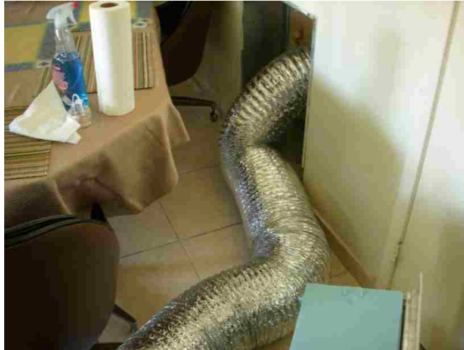
Figure 10. Duct Blaster installed in return register for house #8
