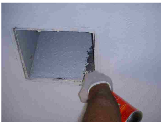
Figure 18. Register sealed neatly using Insulating Foam Sealant in house # 7
