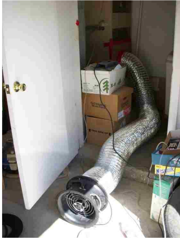
Figure 8. Duct Blaster installed in the air handling unit of house # 7
