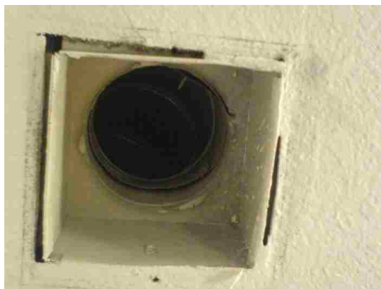
Figure 15. Register opened to do the sealing job in house #5
