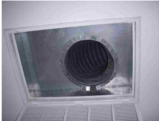
Figure 19. Return register opened to do sealing job in house # 7
