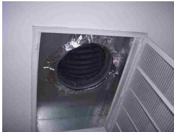
Figure 20. Return register sealed neatly using aluminum tape in house # 7
