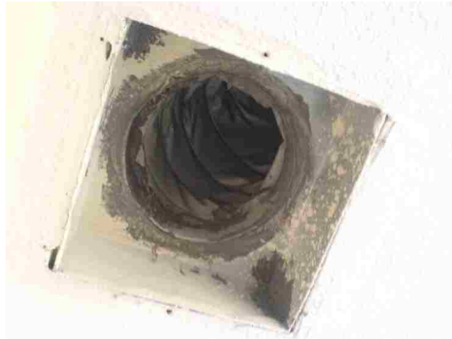
Figure 16. Register Sealed neatly using smooth gray water based sealant in house #5
