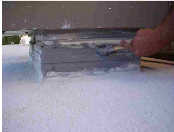
Figure 21. Leakage sealed using smooth water based sealant
