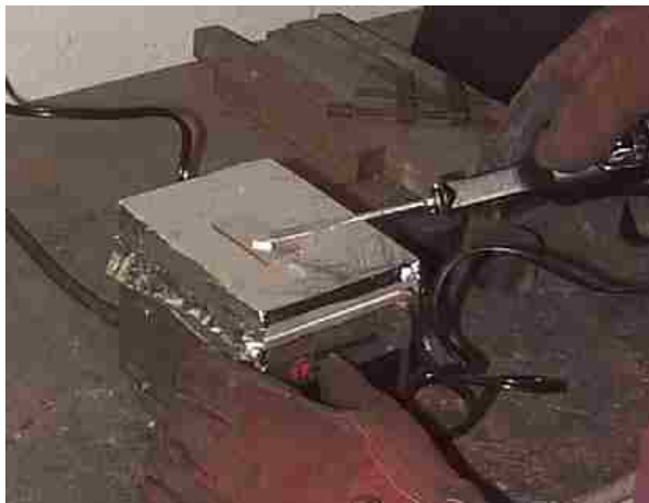
Fig. 34: Spreading S-bond with vibrapeen tool
