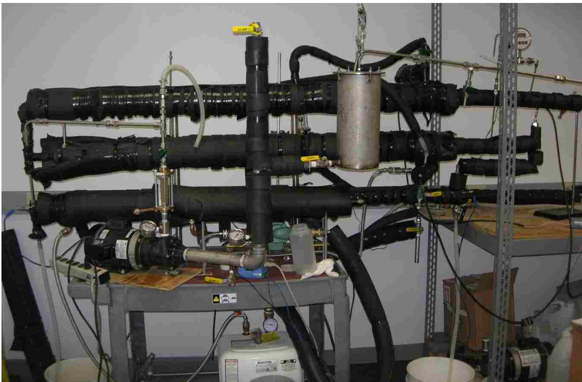
Figure 3: Heat exchanger at Dynalene used for heat transfer tests on spherical nanoparticle nanofluids.
