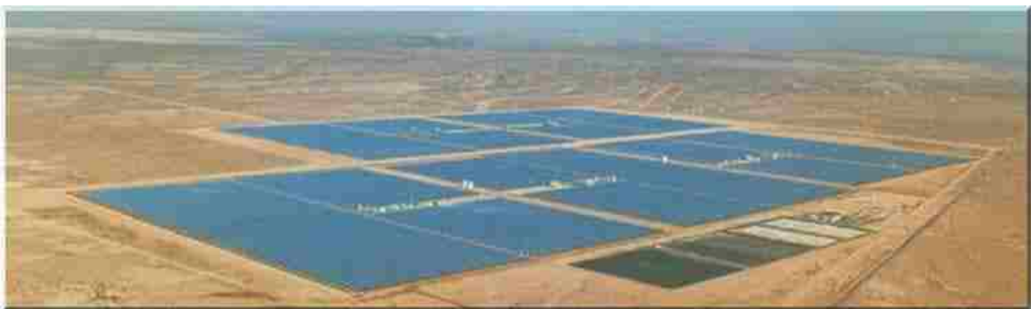
Figure 1: SEGS III to SEGS VII in Kramer Junction, California [1]
