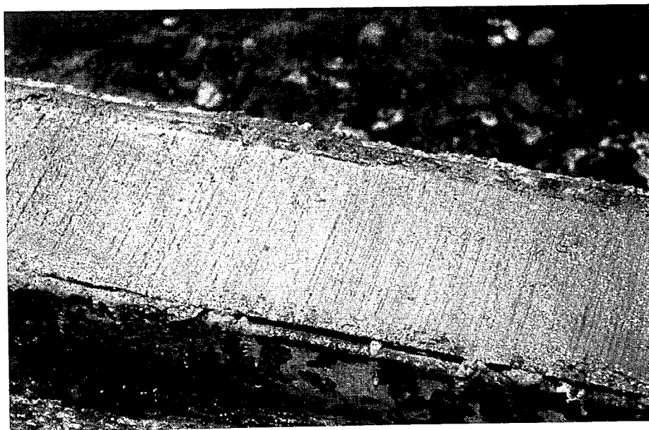
Figure 7-11: Broom Surface Finish
