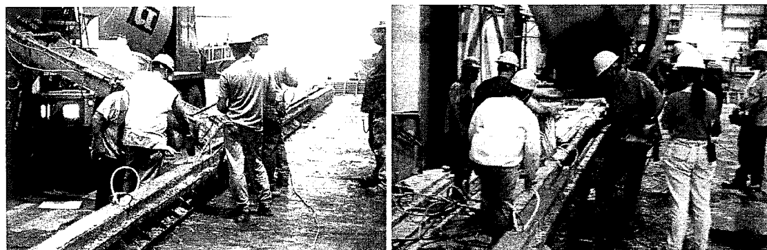
Figure 7-6: Placement of Web Concrete
