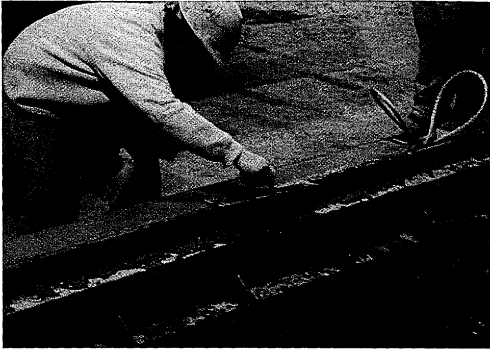
Figure 7-8: Applying a Smooth Surface Finish with a Hard Trowel
