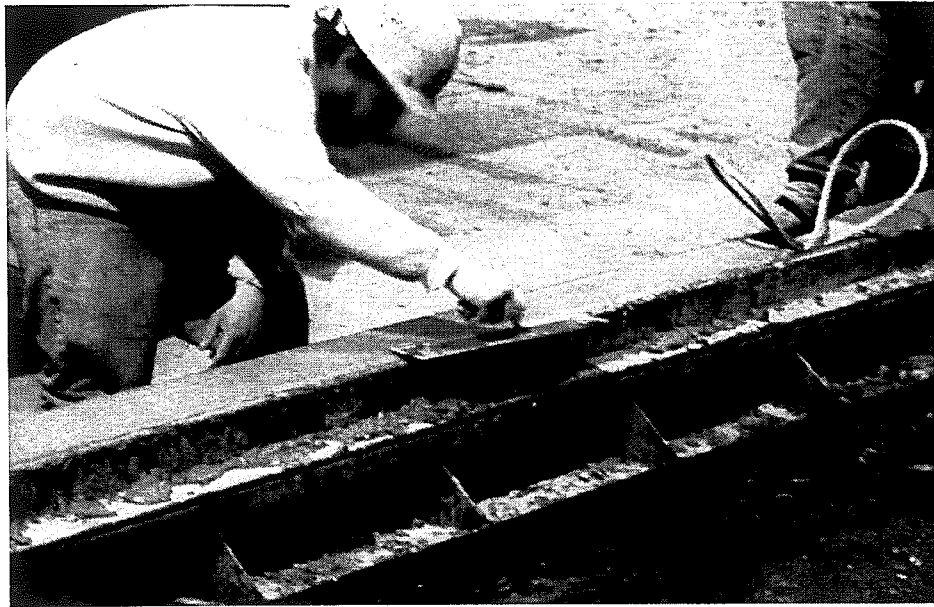
Figure 7-8: Applying a Smooth Surface Finish with a Hard Trowel
