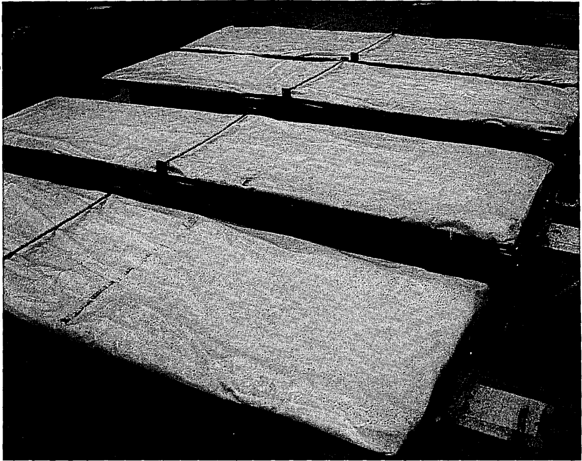
Figure 7-24: Slab Concrete Moist Curing
