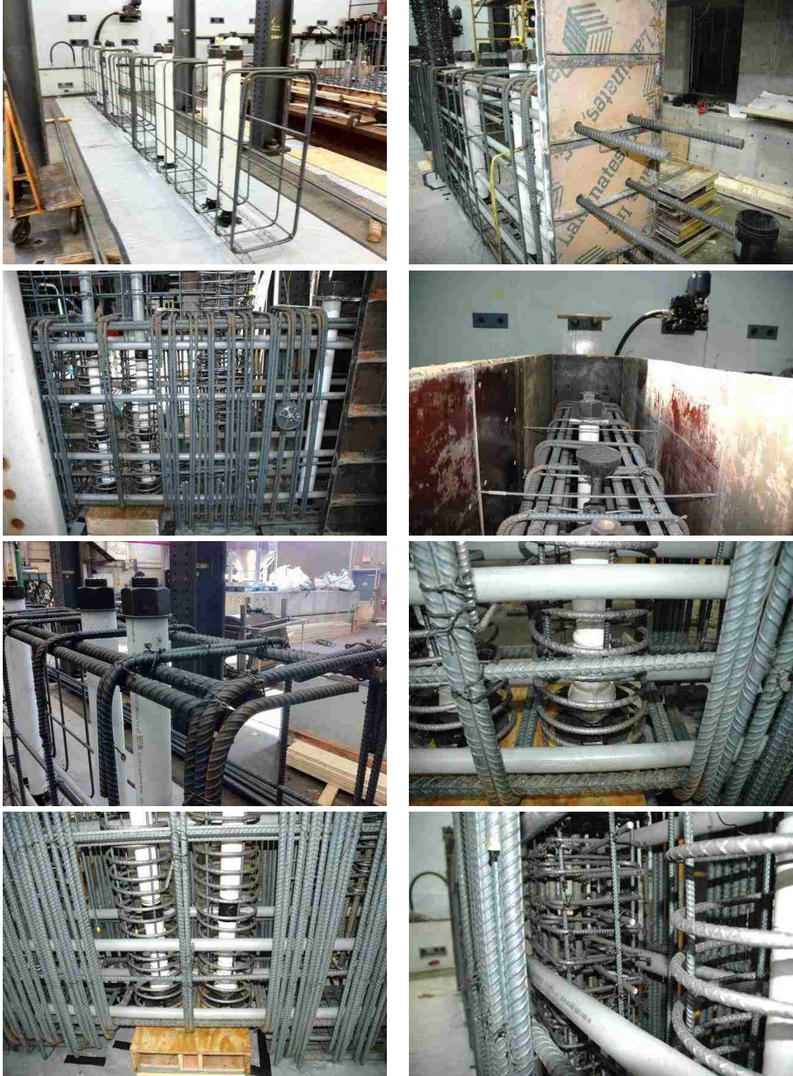
Figure 3-18 Construction photographs of the steel reinforcement cage for the foundation block
