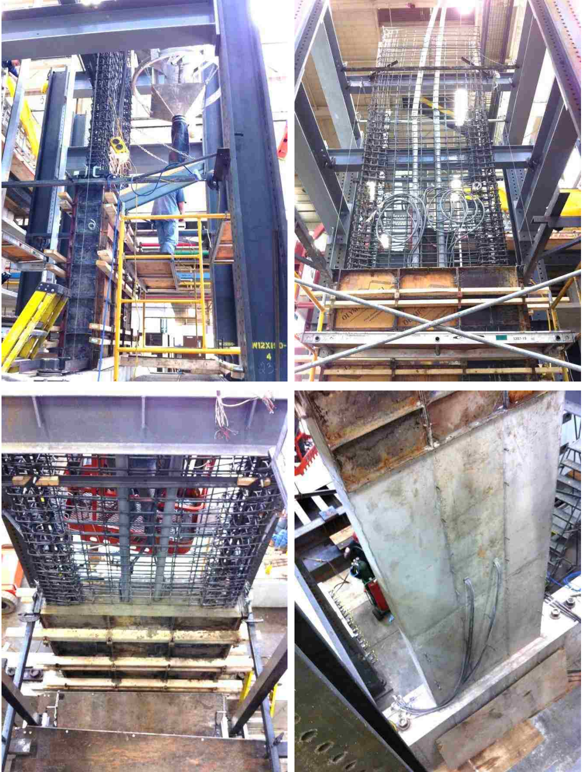
Figure 3-24 Additional construction photographs
