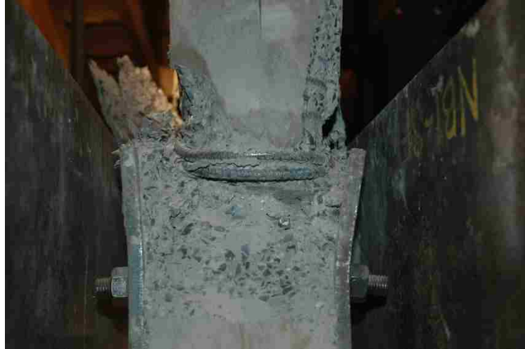
Figure 5-10 - Damage Event 2 - Confinement Failure at Top East Corner of Plate-Confined Panel
