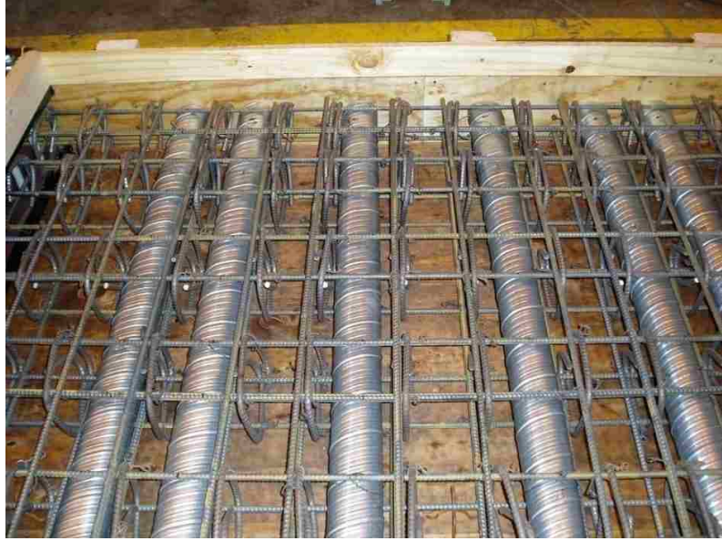
Figure 4-6 - Rebar Cage Detail
