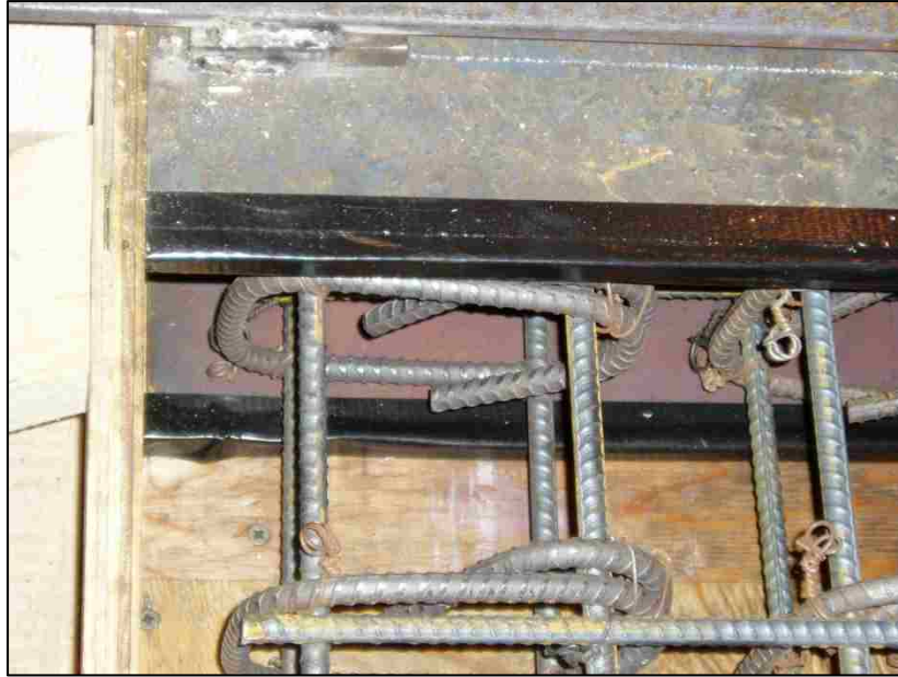
Figure 4-4 - Foam Taped to Confinement Plate for Stiffness Transition
