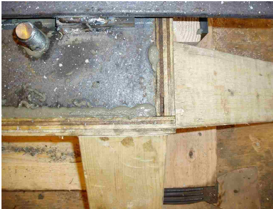
Figure 4-8 - Pouring the Panel
