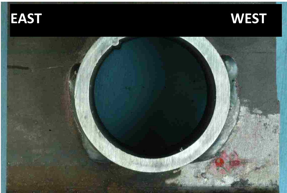
Figure 69. S5-T2 connection cut out, north face
