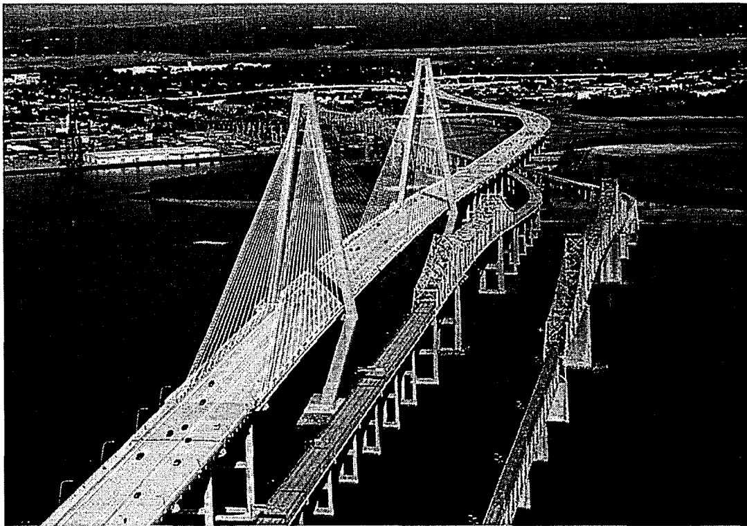
Figure 1.10 View of the Arthur Ravenel Jr. Bridge in South Carolina (Courtesy of http://ravenelbridge.net )
