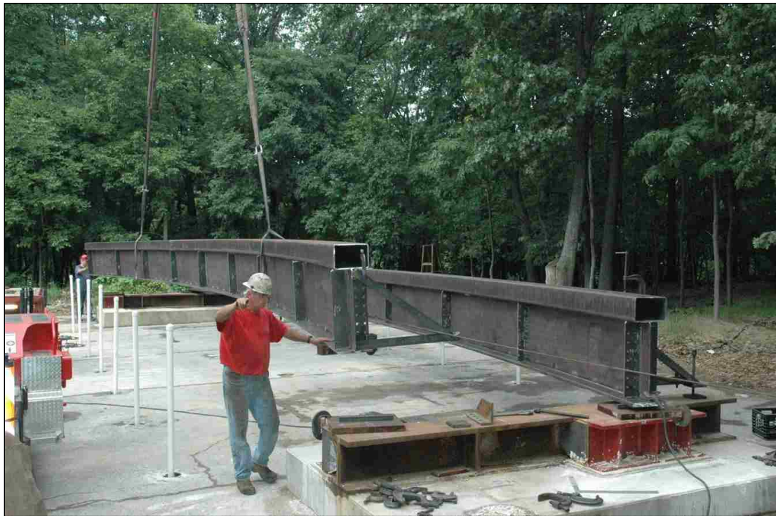
Figure 3.20: Erection of test specimen (Sause et al., 2009)
