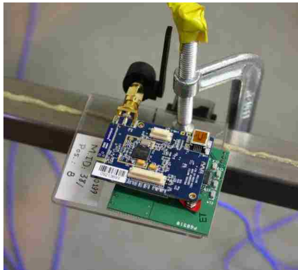
Figure 3.9. Wireless sensor consisting of the SHM-A sensor board attached the an Imote2 processor board, shown mounted on beam at node 8
