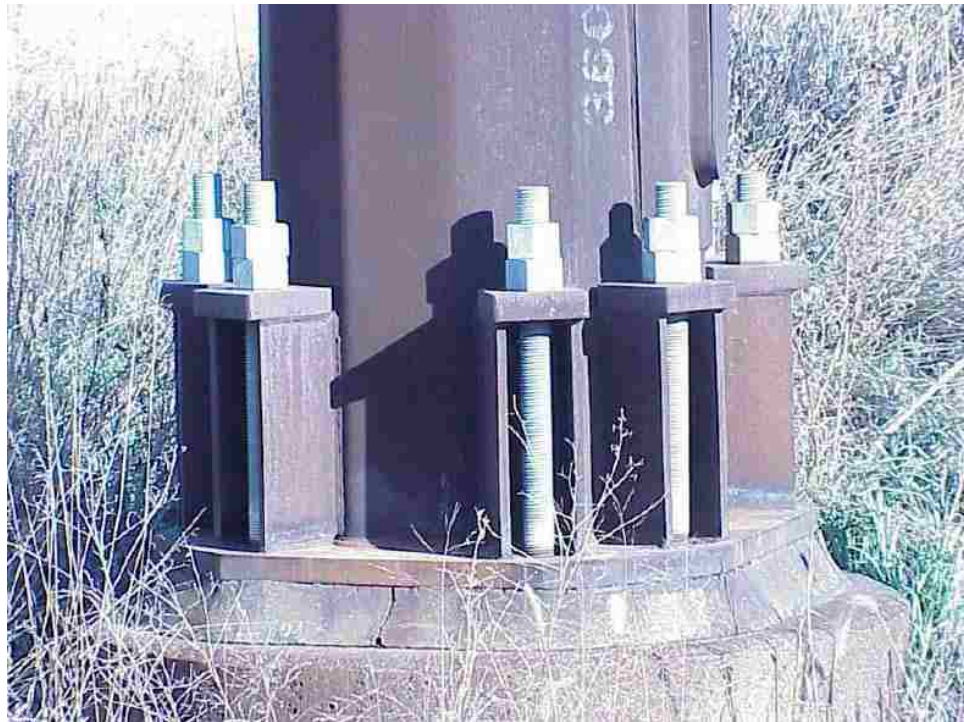
Figure 6. Stool base connection detail ( reprinted from Dexter, 2004 )
