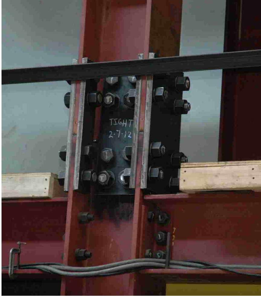
Figure 4.37- Photograph of bracing frame repair
