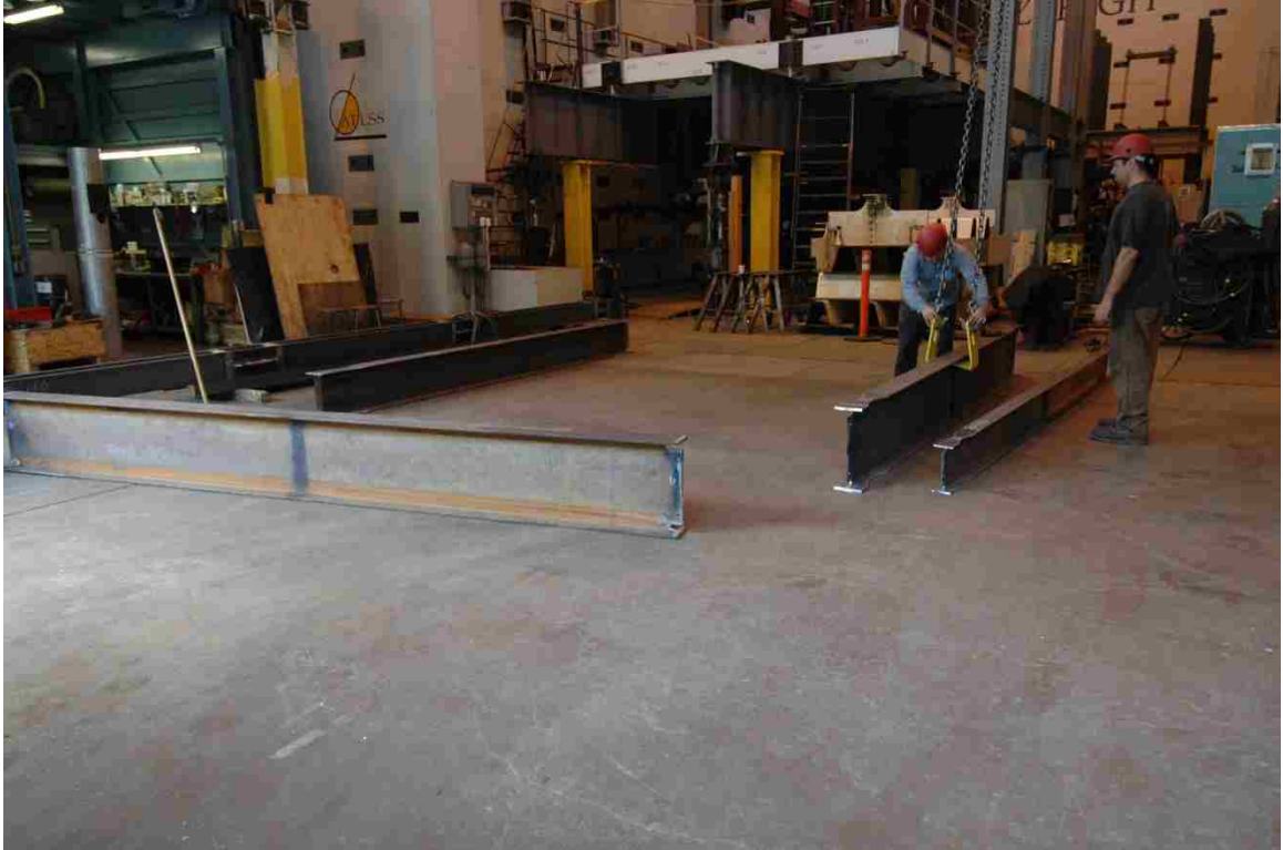
Figure 4.11 – MRF Being Assembled
