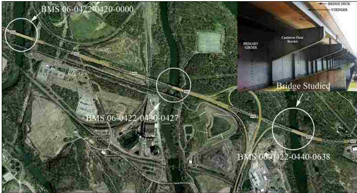
Figure 2-1: Bridge location (Google Maps 2010) and view of bridge looking east from Abutment 1
