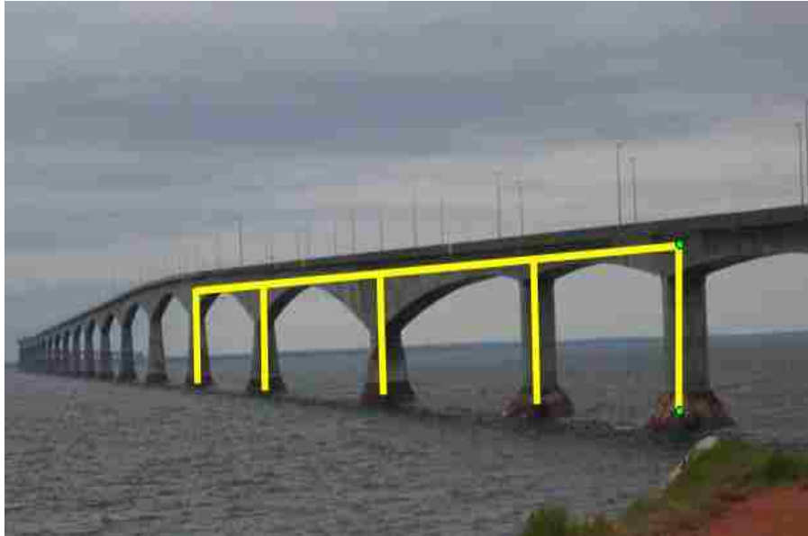
Figure 2.4a Application of Column-Beam Frame on a Bridge
