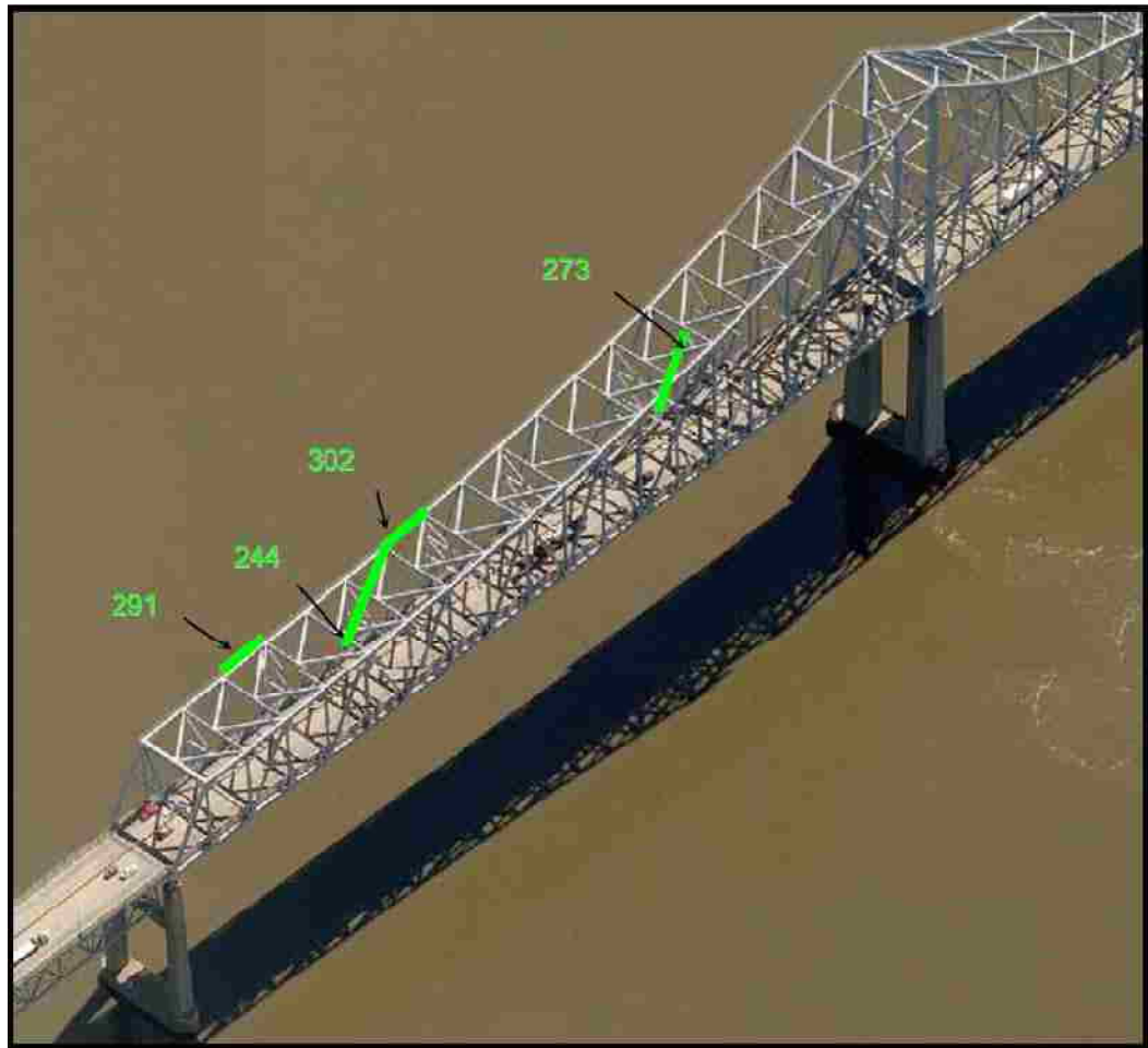
Figure 5.3 Photographic view of Pennsylvania back span looking upstream showing instrumented truss members (green = upstream; yellow = downstream) (From Hodgson et. al, 2008)
