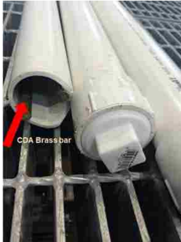
Figure S1. Pipe rigs with CDA brass bar simulating distribution system with premise plumbing
