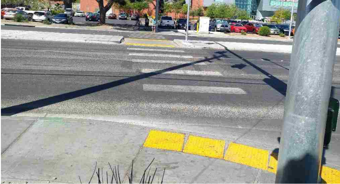
Figure 9. Typical crosswalk markings
