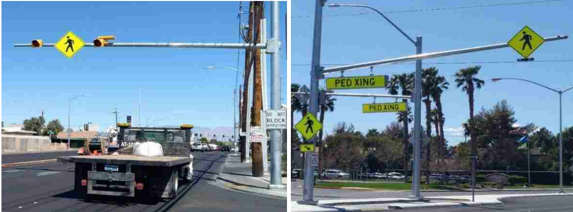
(a). Circular Rapid Flashing Beacons (CRFBs) (b). Rectangular Rapid Flashing Beacons (RRFBs)
