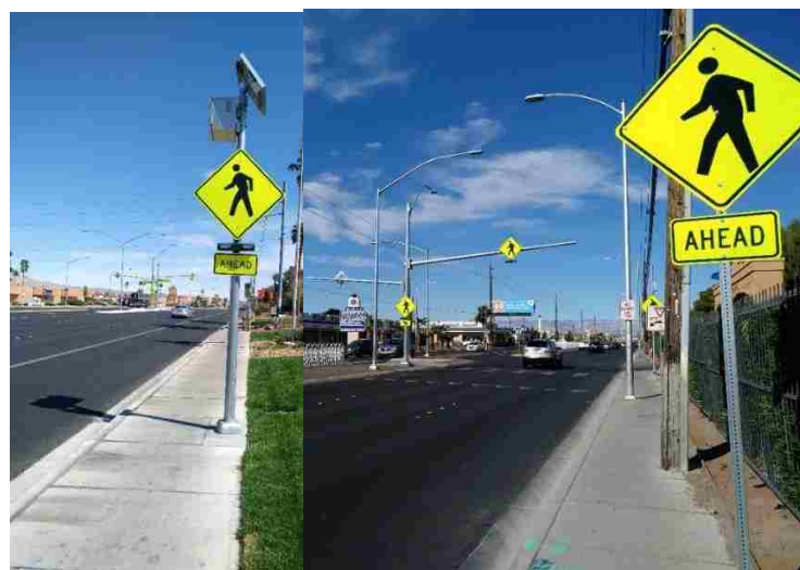
Figure 14. Advanced pedestrian crossing signs with and without flashers
