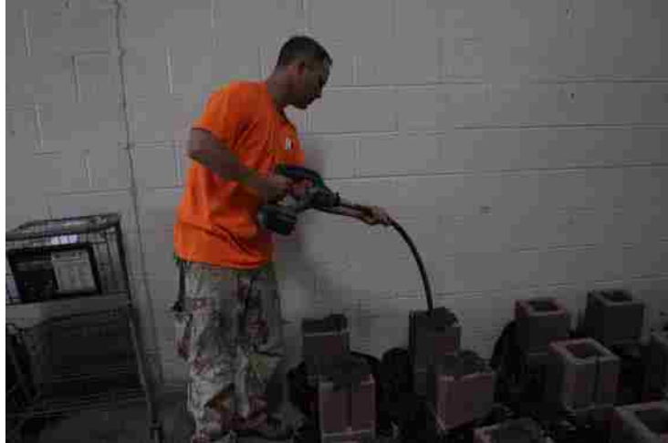
Figure 4- Consolidation of Grout
