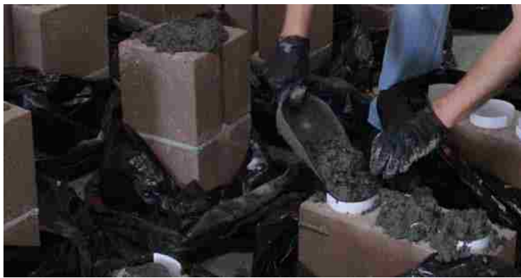
Figure 3- Placement of Grout
