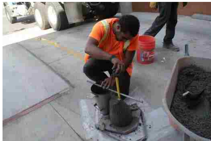
Figure 7- Slump Measurement by ACI Technician
