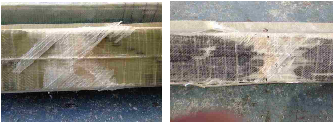
Figure 15: Delamination of plies in shear webs & compression flange
