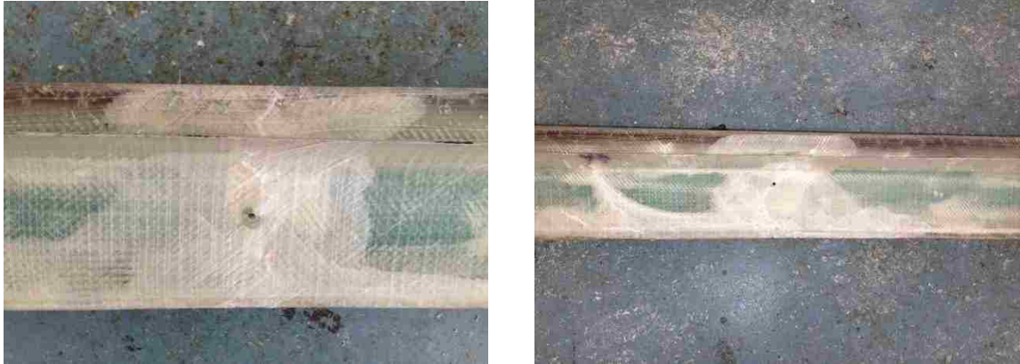
Figure 14: Crack passing through rivet hole
