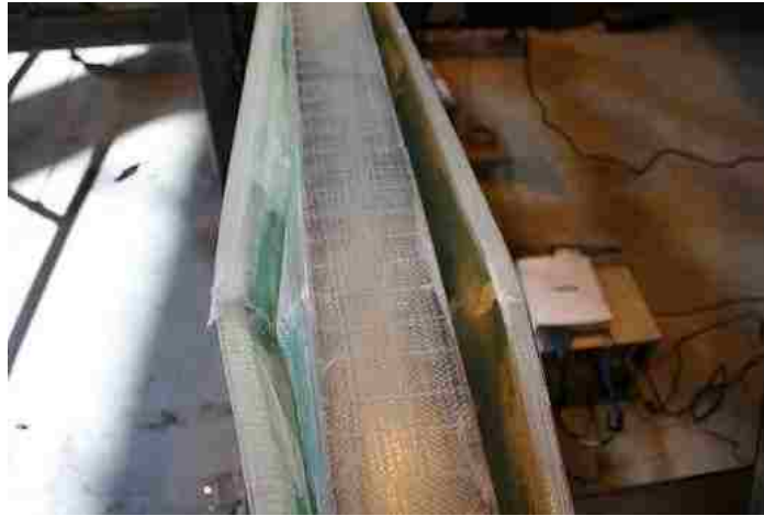
Figure 13: Debonding of shear webs
