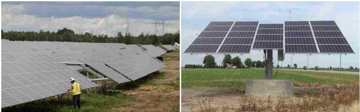
Figure 1.1: Examples of solar panels installed in a solar farm (adapted from The Globe and Mail) and in a rural area
