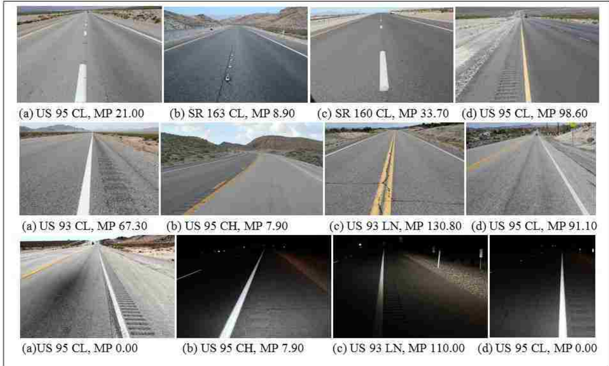
Figure 4.3. Photos of Striping Performed by In-House and Private Contractors under MBC and PBC Methods
