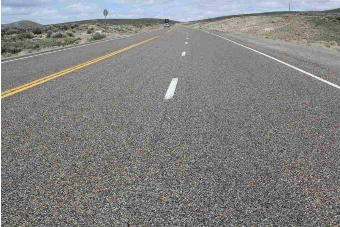
Chip Seal, State Force, US 93 EL County 2011
