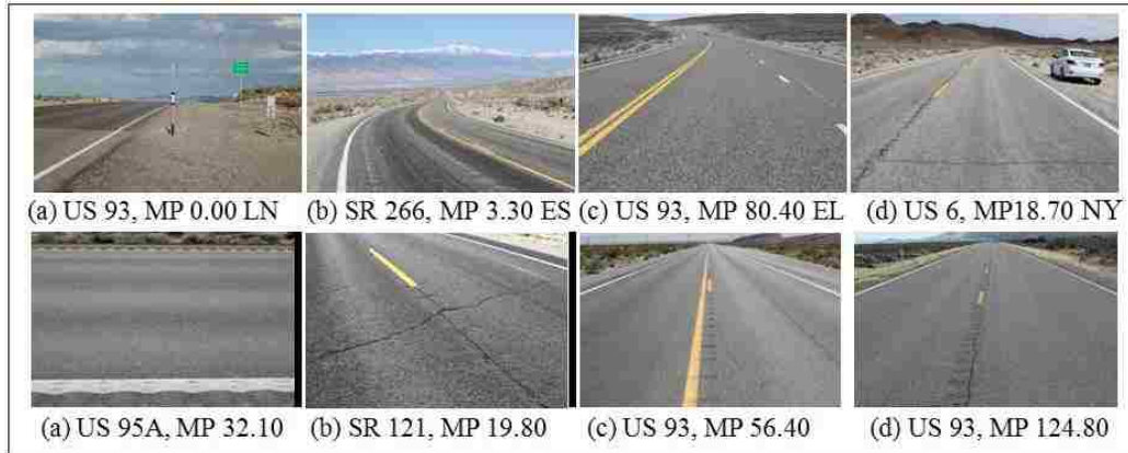
Figure 4.2 Photos of road sections with chip seal performed by In-House and MBC methods.
