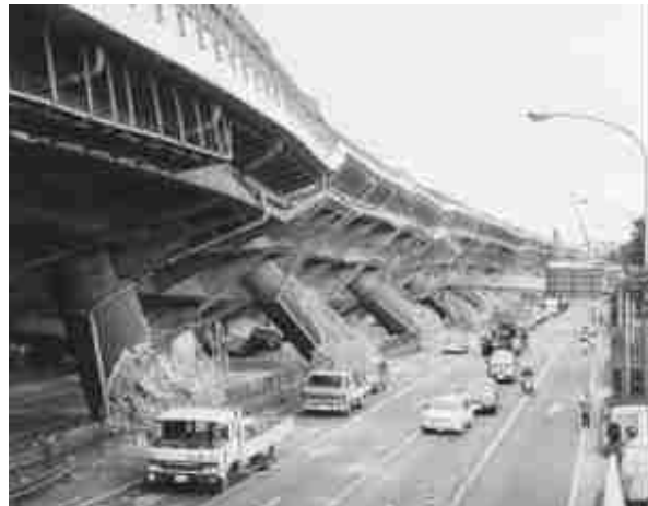
Figure 2-11 Collapse of Hanshin Expressway due to substructure failure (Chen and Scawthorn 2003).
