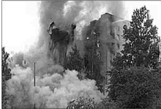
Figure 1-2 Collapse of St. Petersburg Apartment Block ( Russian apartment block collapses.2002 )
