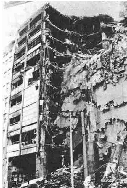
Figure 1-4 Collapse of Katrantzos Sports Department Store (Papaioannou, 1986)
