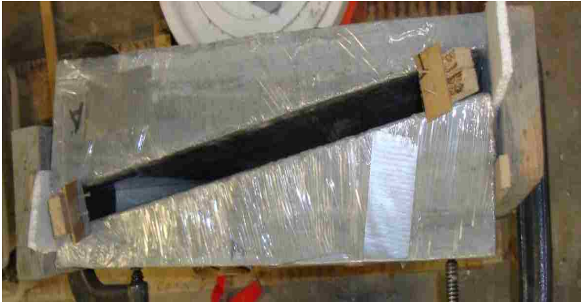
Figure 13.4: Formwork set up for hyperbolic paraboloid shells
