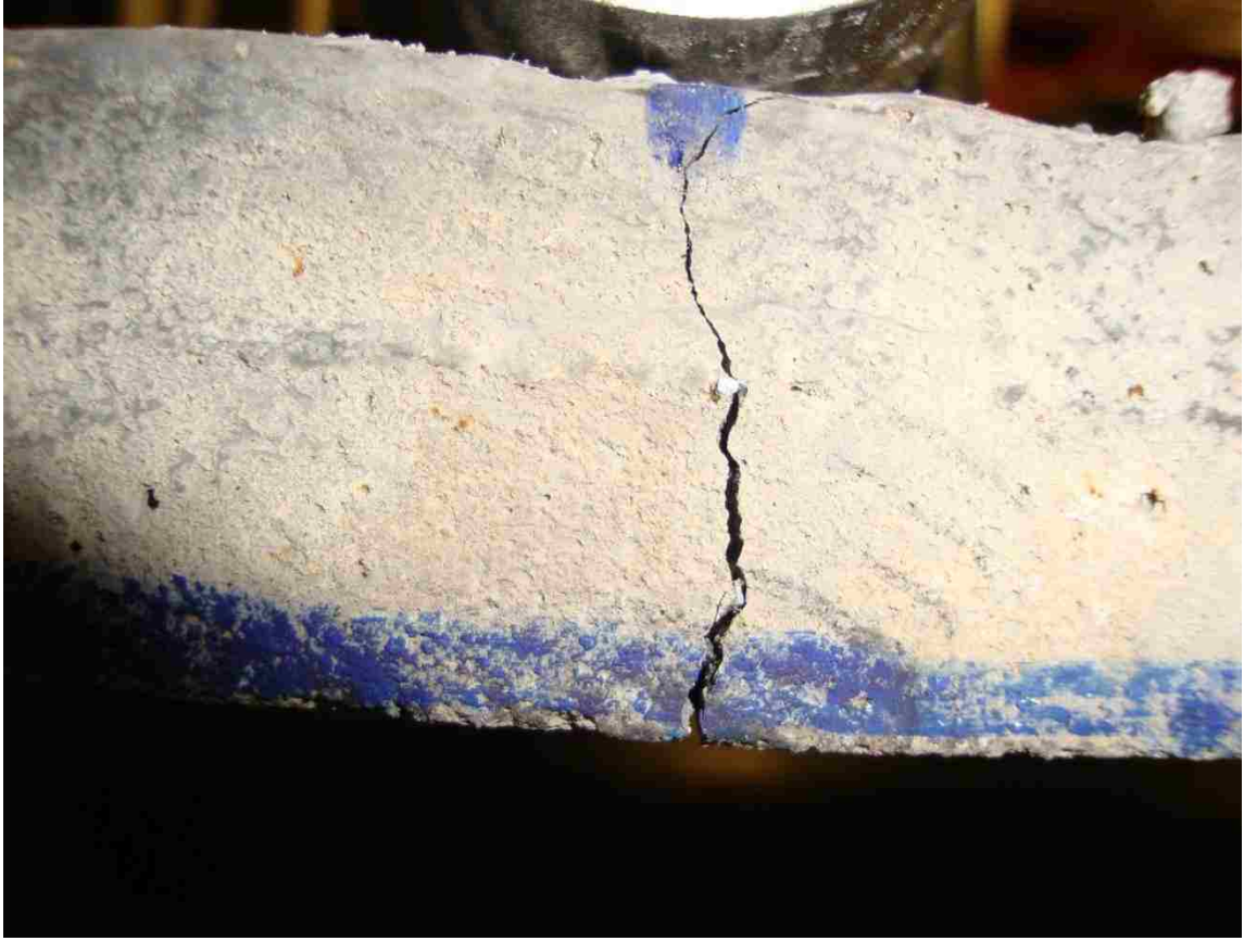
Figure 8.1.13: Failure patterns for long span 1% HSSFRC rectangular plates under transverse line load
