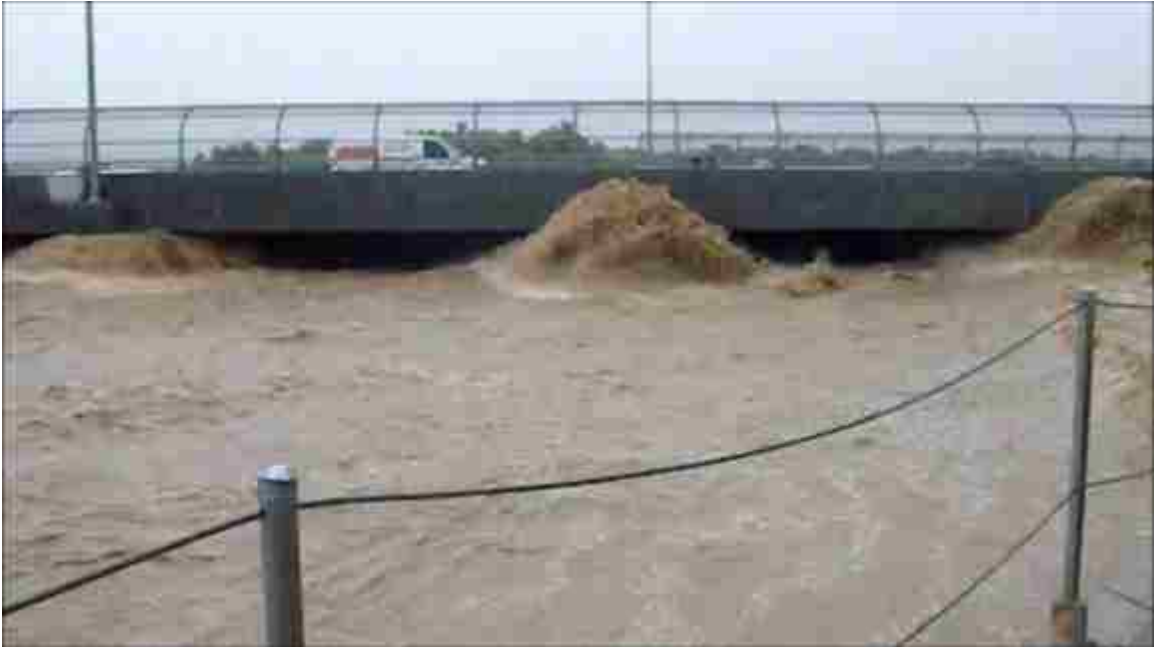
Figure 1. Duck Creek flood channel, Las Vegas metropolitan area. (Provided by CCRFCD, 2013)
