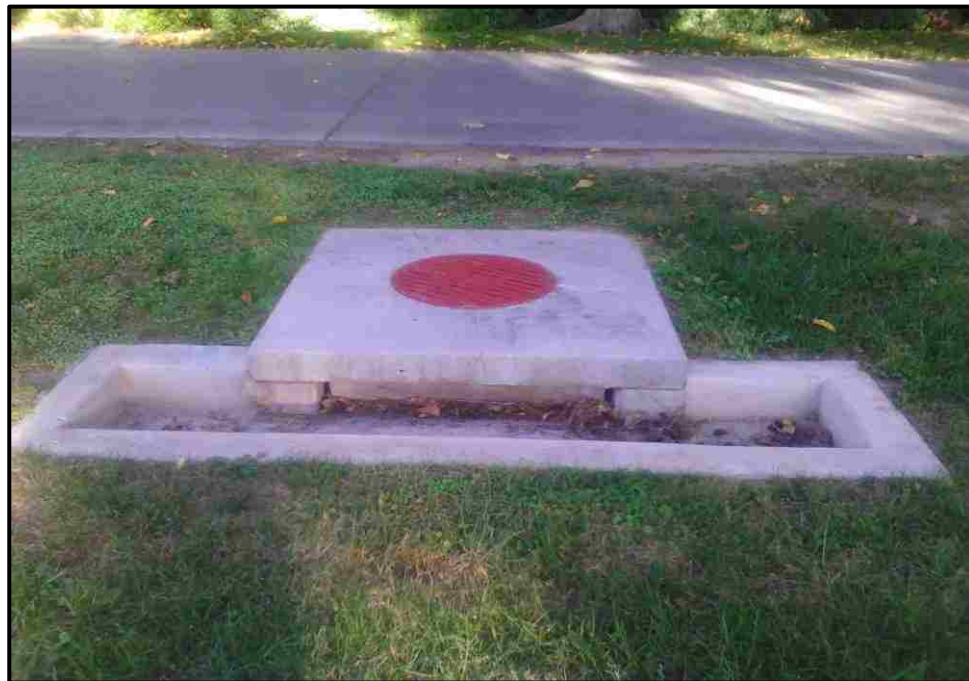
Figure 3.1-4: Storm drain inlet at the East Mall area
