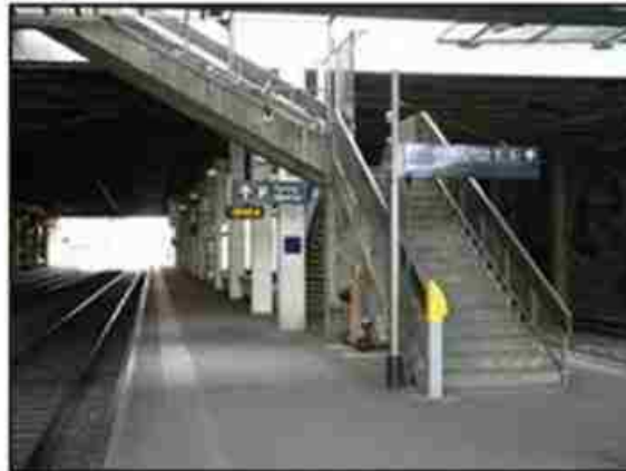
Access to the Platform in Angers-St-Laud
