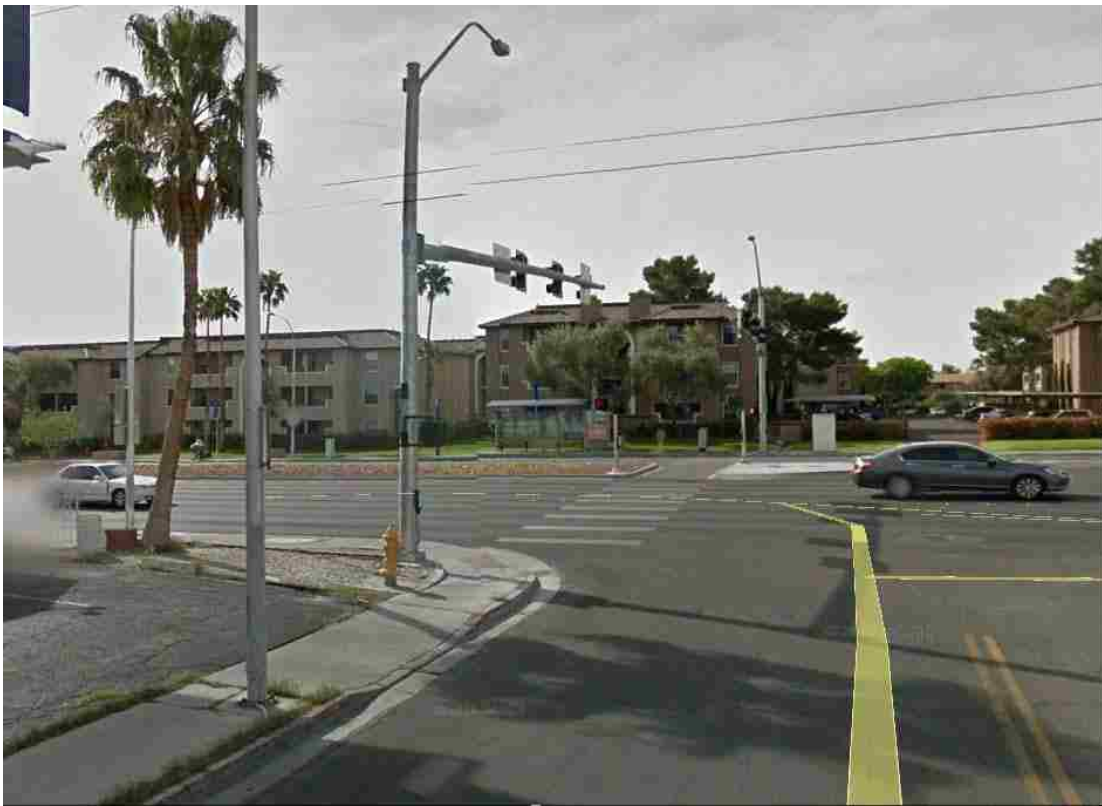
Figure 3-9. View of PHB System (Facing South on S. 15 th St., Google Map)
