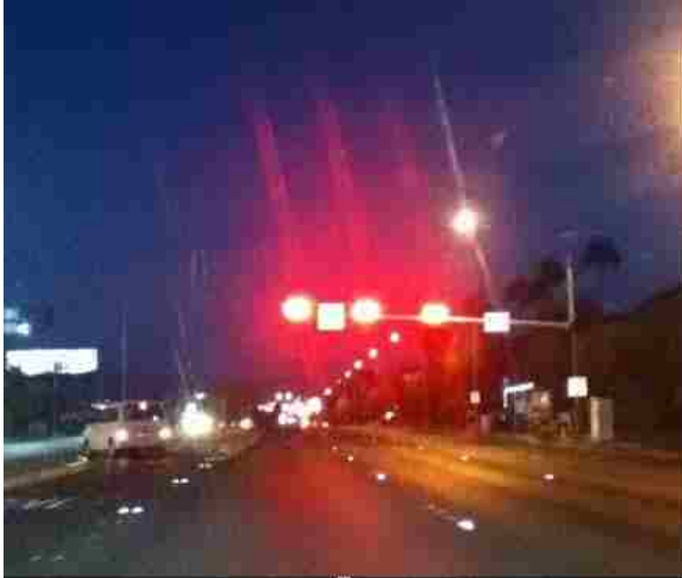
Figure 3-13. View of Activated PHB System at Night
