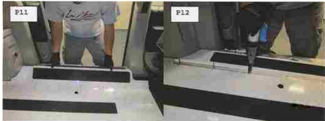
FIGURE 3- 7 INSTALL THE SIDE PANELS
