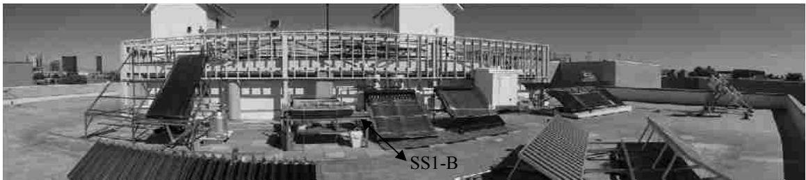
Figure 2.2 Northern view as seen from the parapet
