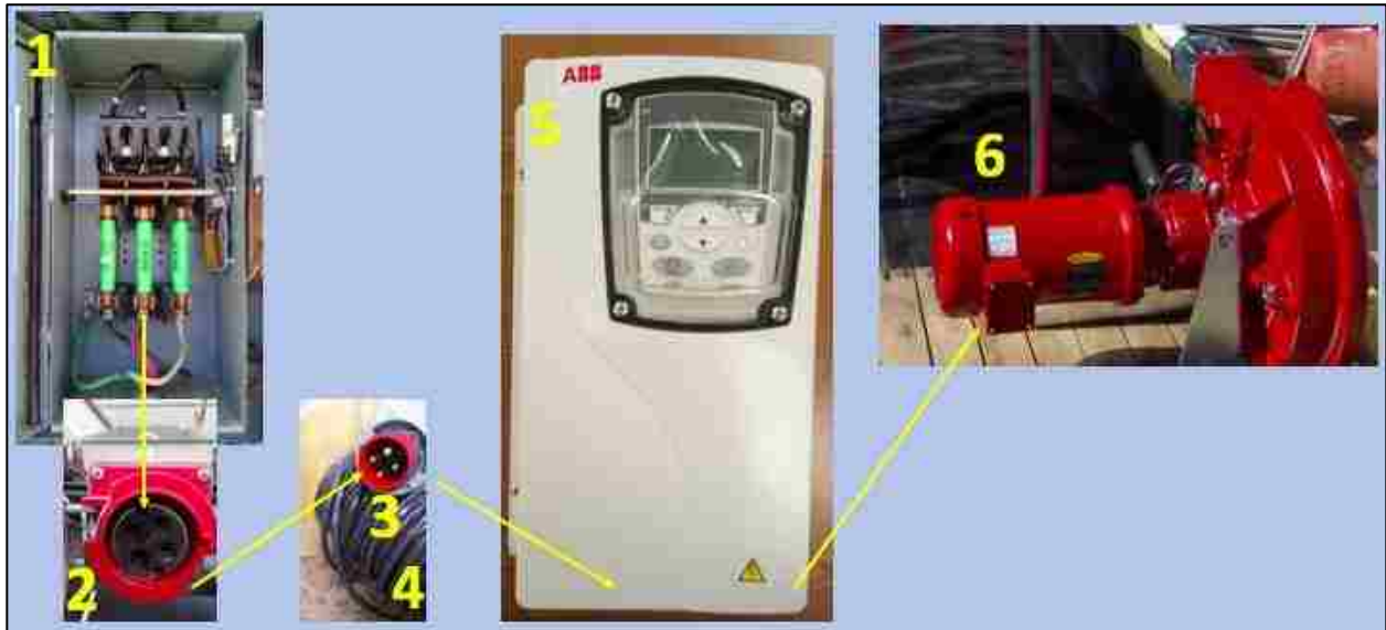
Fig. 13. Simplified High Voltage Power System
