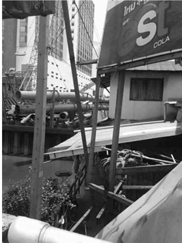
Image 6.16. Demolition of dwelling spaces along Khlong Lat Prao. August 2016. Own Image.
