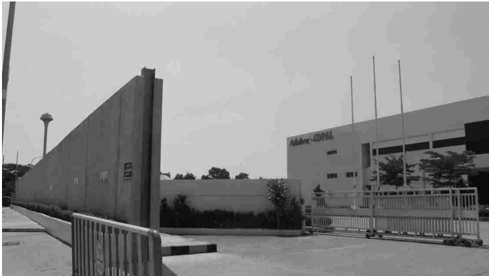
Image 5.2. Floodwall in front of Nidec-Copal company. Industrial estate near Ayuthaya. Own image.
