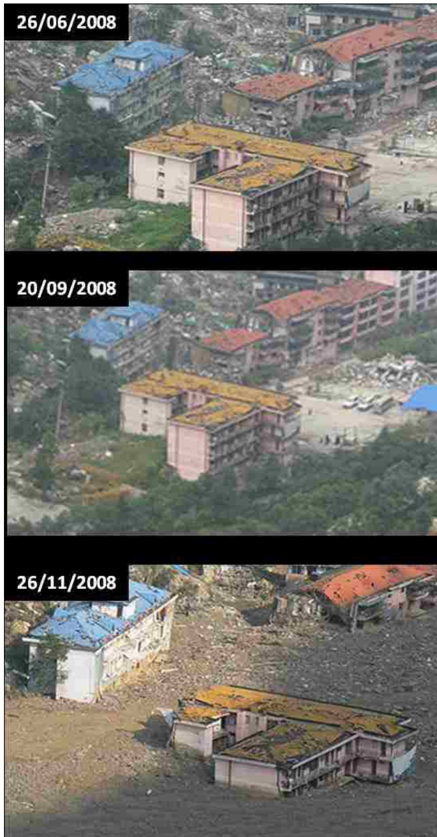
Figure 5.2: Initial photograph collection of Beichuan town, illustrating the temporal changes in sediment aggradation.
