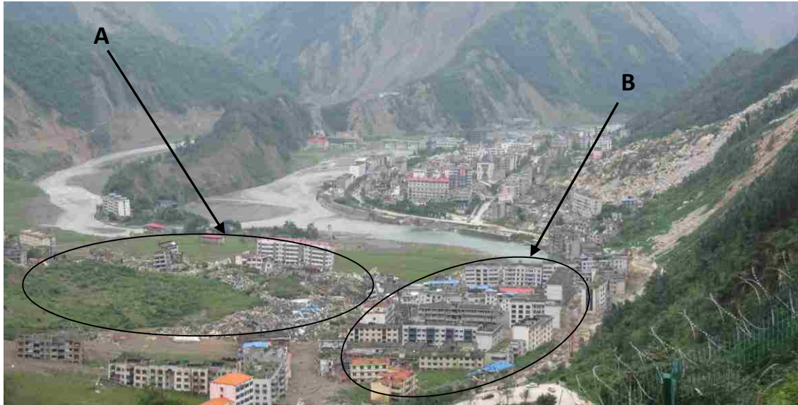
Figure 2.1: Photograph showing the differential impact upon the level of building collapse between two different areas of Beichuan Town. A shows an area where almost all buildings collapsed, whereas B shows a different area where most buildings remained standing.
