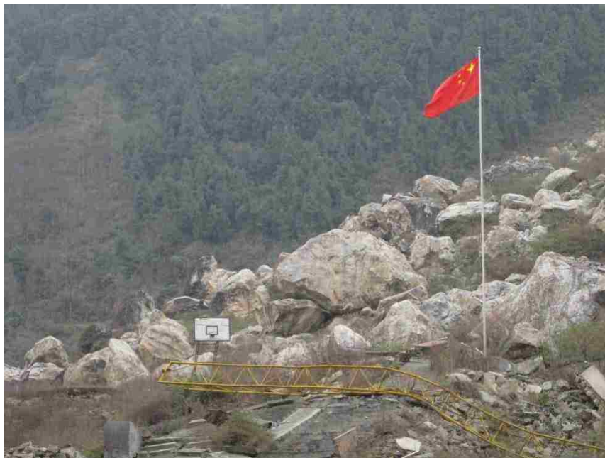
Figure 4.3: The school flag and basketball hoop were all that survived the rockfall which crushed Maoba Middle School. (Source: Authors own photograph)
