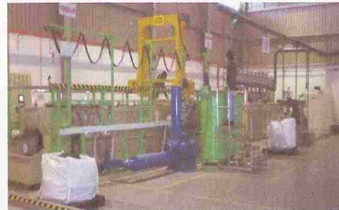
Plate 2.13: An e-waste recovery plant. (Source: Reclaimtek (M) Sdn. Bhd.)
