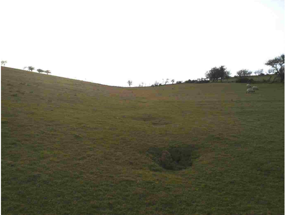
Figure 3.5: View upstream of the channel from the sump showing drain excavations as a result of the broken drainage pipe.
