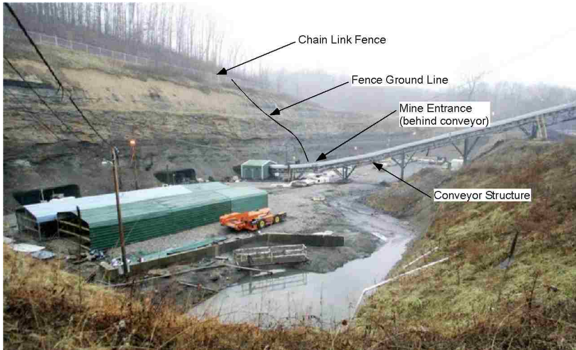
Figure 2-2 Sago Mine with fence ground example.
