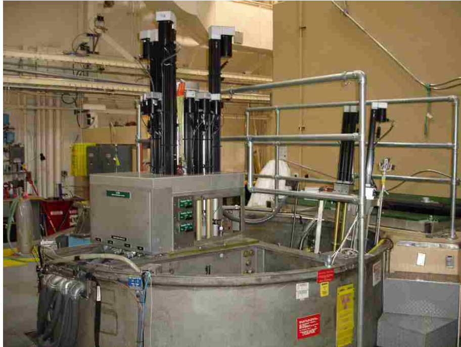
Figure 1.3: Top of the ACRR Tank.
