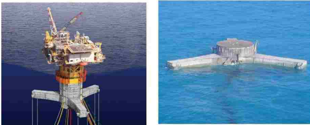
Figure 52: Chevron’s Typhoon TLP - pre and post hurricane Rita condition (From DNV Report- 44814183)
