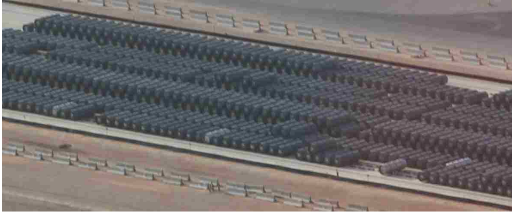
UBC Storage Pad at the UUSA Enrichment Facility in Eunice, New Mexico
