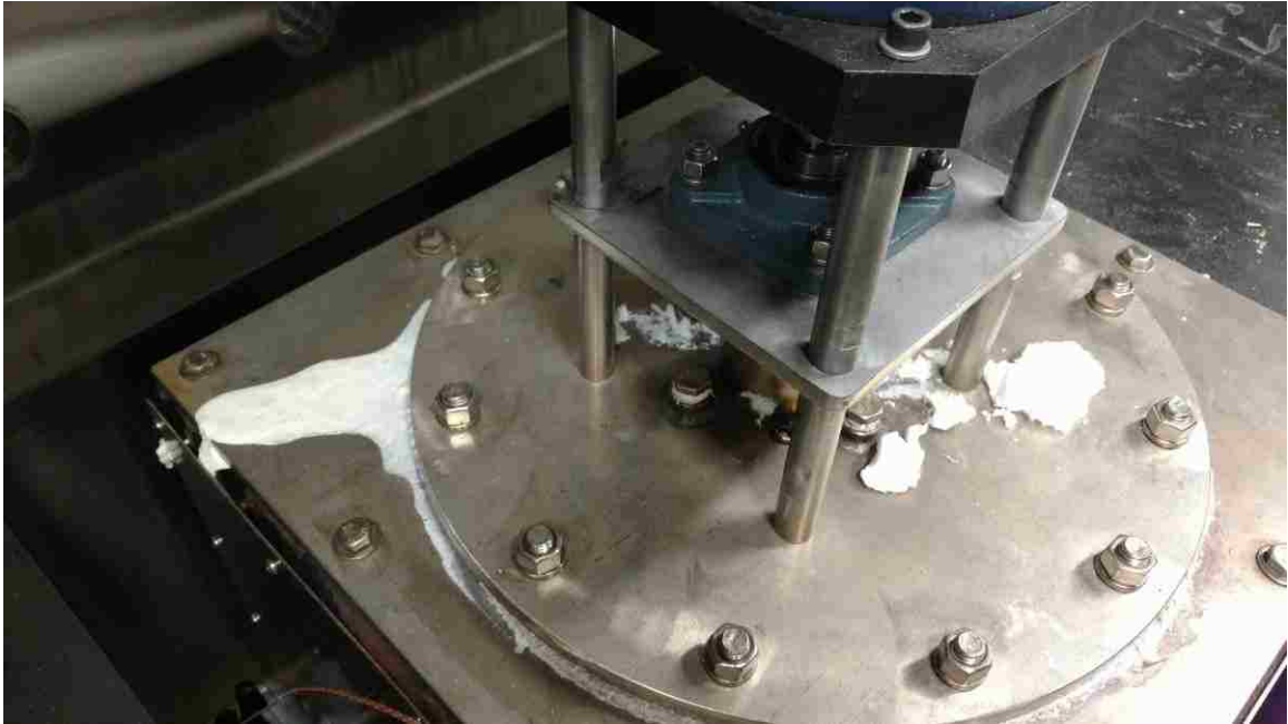
Figure 2-29 Melt tank leak
