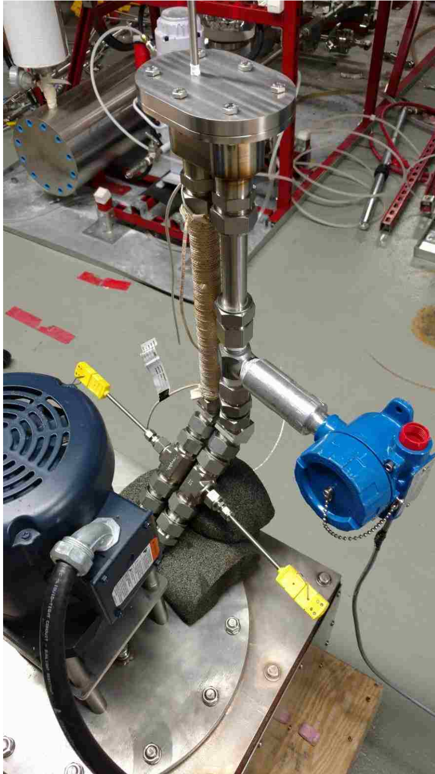
Figure 3-14 Loop of Assembled Tubing and Fittings
