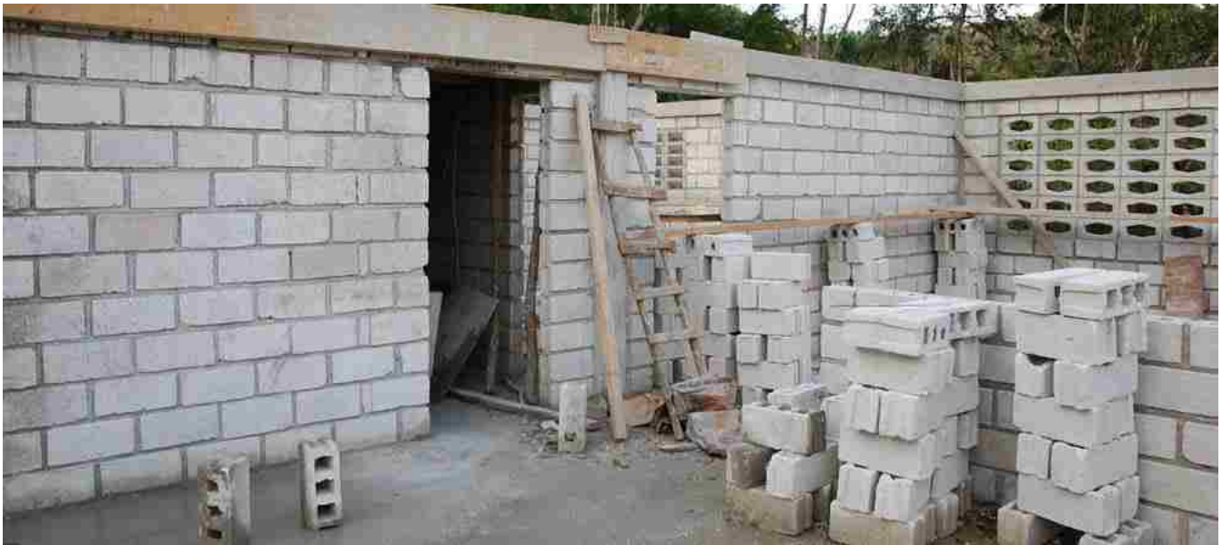
Fig. 4.6: Concrete Block Construction
