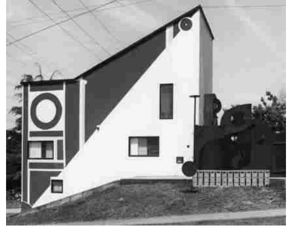
8.4 Reichert house-studio facade. (Robert Reichert Collection, UW Libraries Special Collections UW40099).
