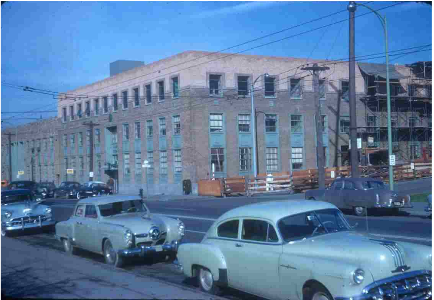
0.6 Kodachrome slide of Seattle Labor Temple, 2800 1st Avenue, taken by Reichert, c. 1955, with the annotation, “I did 3rd floor add’n.” The brick color of the new addition is clearly differentiated from the lower floors. The original building dates from 1942 and 1946, designed by McClelland and Jones; the addition is credited to Harmon, Pray and Dietrich, 1955. (UW College of Built Environments Visual Resources Collection).
